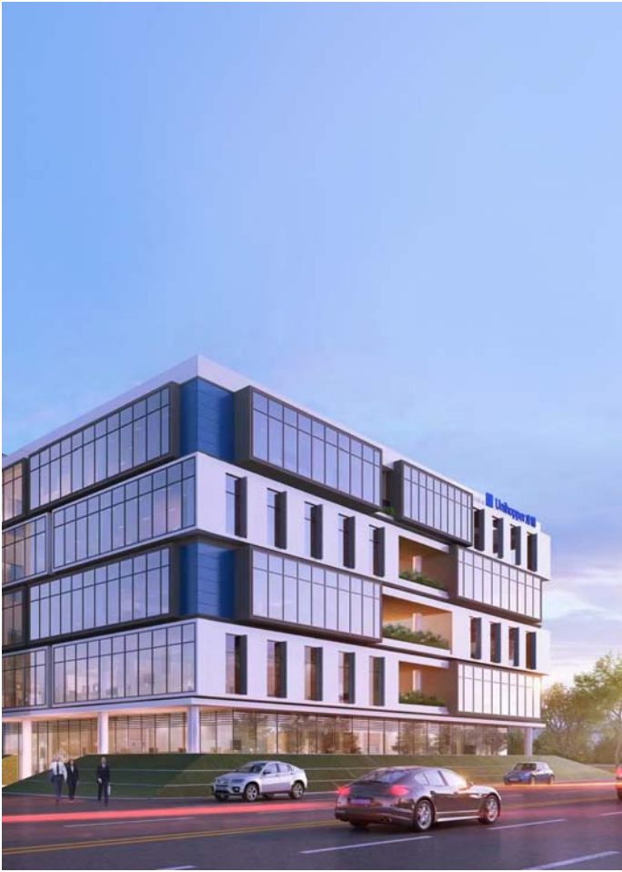
Unihopper R & D Building
